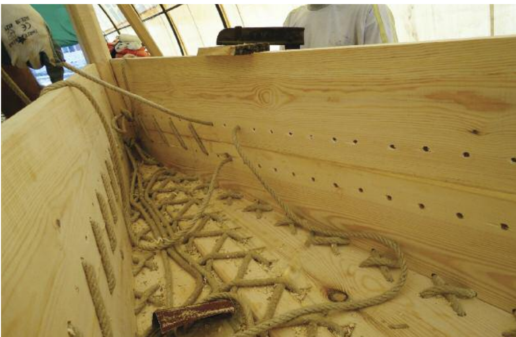
Fig. 3 Puncturing and stitching the hull.
