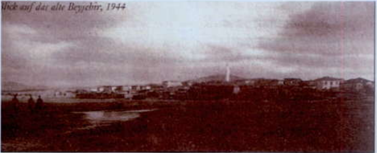
RESİM 11 - BEYŞEHİR / FIGURE 11 - BEYSEHIR
