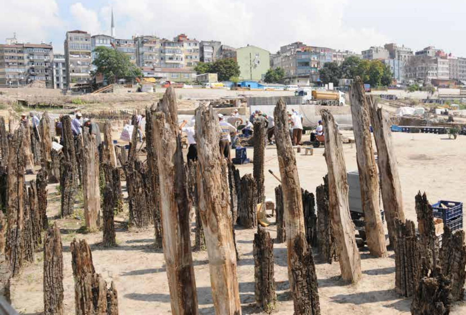
Fig. 6: Wooden pier footings.
